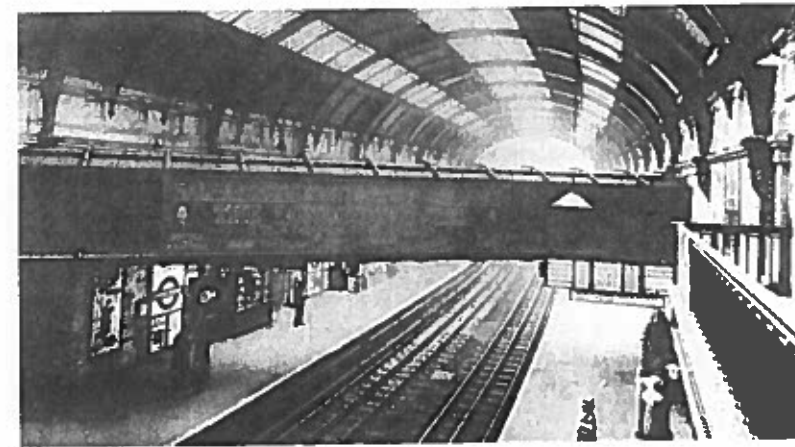
Remembered by the over-sixties. The roofed Underground station at Sloane Square in the 1920s with the Westbourne river flowing through its pipe above the lines. The roof was destroyed in the November, 1940 bombing. Another illustration from Chelsea Past.
