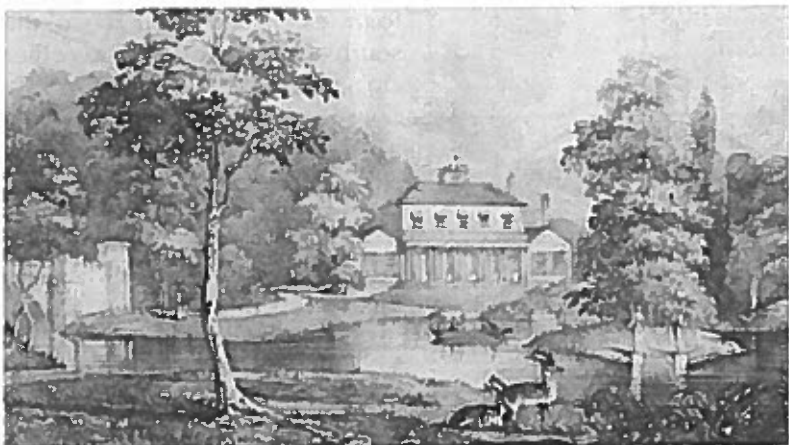
South view in 1829 with the mediaeval style bridge on the left. (Royal Borough of Kensington and Chelsea Library Services)
