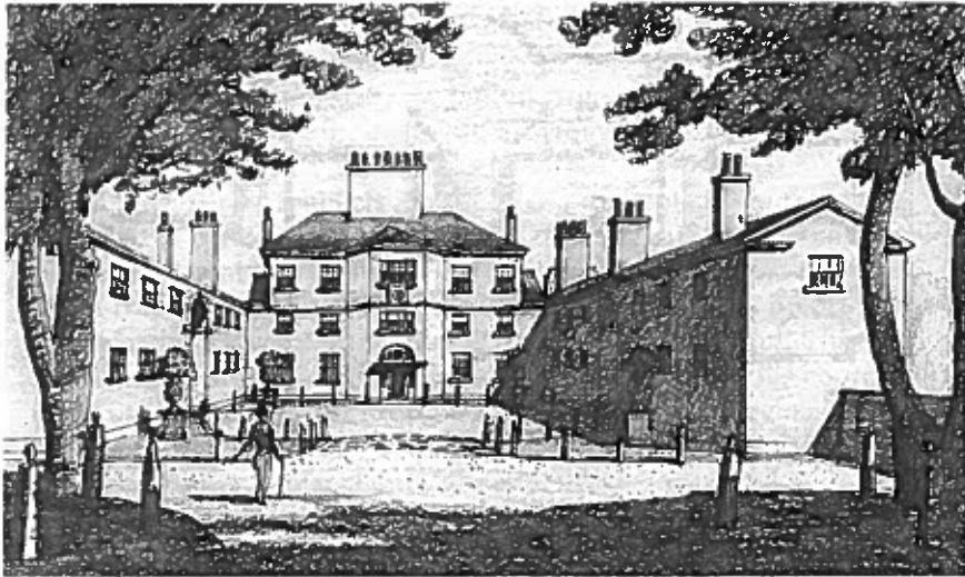
Sketch view of the Entrance courtyard as built by Henry Holland.
