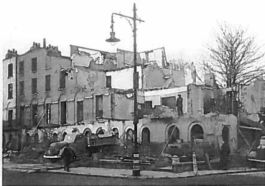
Demolition of the houses in the King's Road from 264 onwards c.1957. Mike and his family lived at no. 282 in the 1950s.
