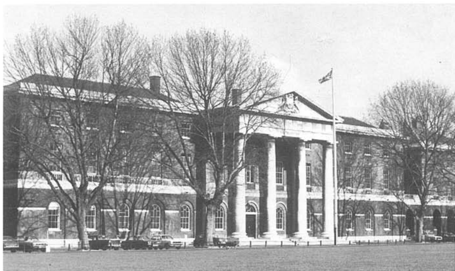
The Duke of York's Headquarters (originally the Royal Military Asylum for the Children of Soldiers of the Regular Army). Architect, John Saunders, 1801-1803. (Photograph by courtesy of Donald W. Insall and Associates, architects.)
