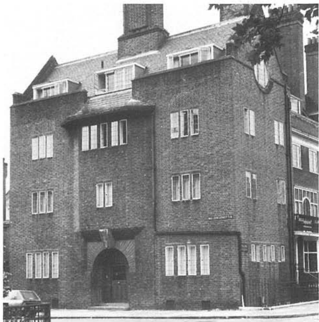
Mallord House, Mallord Street. Ralph Knott, architect. See page 41.
